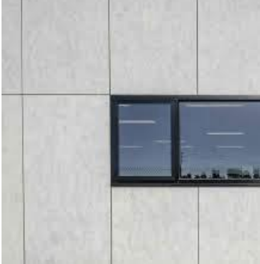
4 COMPRESSED FIBRE CEMENT CLADDING TYPE 3 WITH POWDER COATED WINDOW FRAME C3
